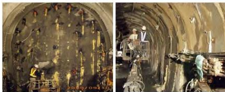
隧道開挖瓦斯洩漏封堵
